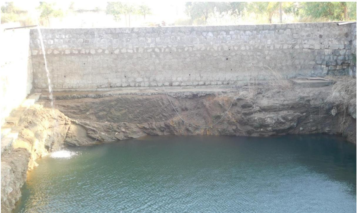
Artificial roof top rain water harvesting pit
